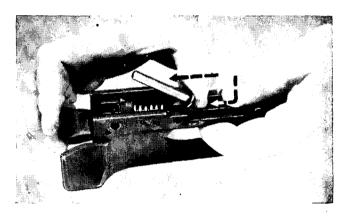
Figure 52. Replacing the sear carrier (second method).
