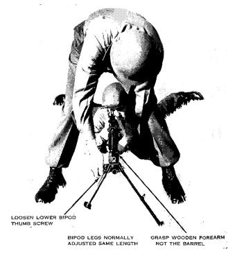
Figure 135. The coach adjusts the bipod legs.
