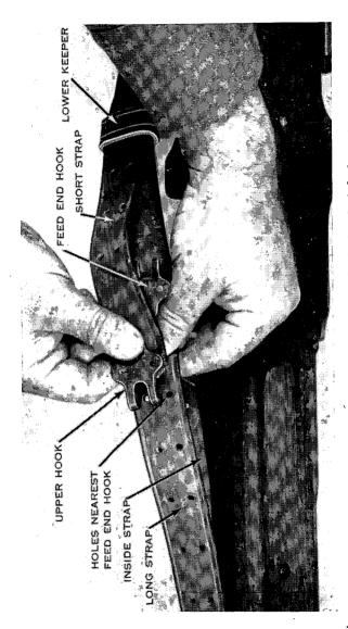
Figure 102. Engaging the upper hook to the feed end of the long strap.
