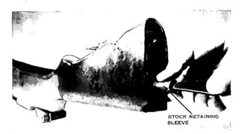
Figure 65. Removing the stock retaining sleeve.
